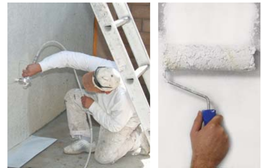
The Bioni Hygienic Food system can be sprayed or applied by roller.
